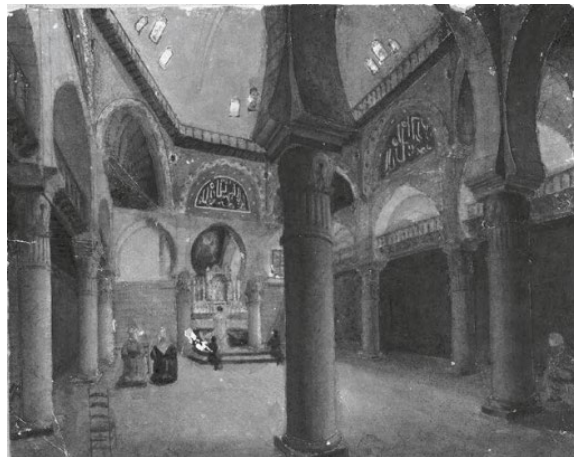
Fig. 3. The prayer hall of Ketchaoua Mosque before 1832, depicted by Charles Desprez, a scanned painting from the National Library Archives in Algeria. (Source: Amal Belala, 2019).
